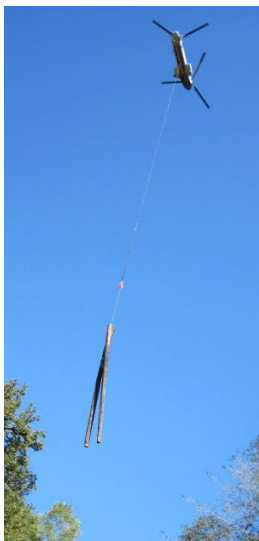
A helicopter places logs in Little Fall Creek.
