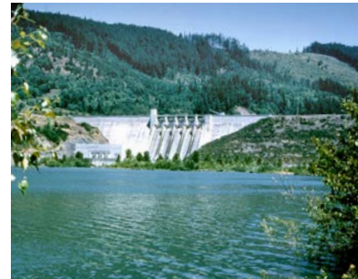
Lookout Point Dam near Lowell.
